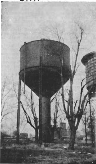
Water tower coated inside and outside with NO-OX-ID. Long lasting reliable protection from rust.
